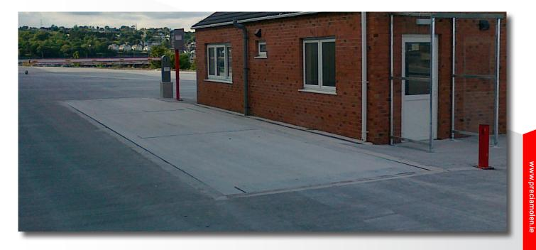
From the world leader in weighbridge technology the Precia Molen VS210CS low profile in-ground or pitmounted weighbridge offers a robust and long lasting, yet cost- effective, road vehicle weighbridge. Designed to operate in the most arduous environments the structure provides unparalleled flexibility for all vehicle weighing applications. Ideal for installations with limited space the VS210CS can accommodate traffic manoeuvring in any direction across the flush platform.
